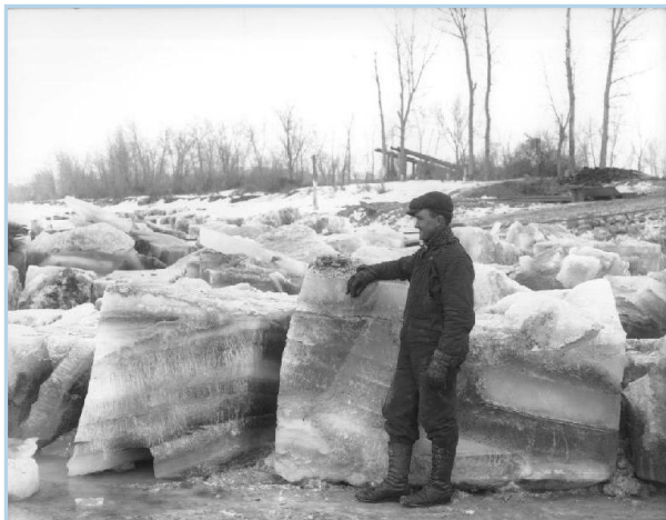
Ice blocks removed from Yellowstone River during construction of Lower Yellowstone Project
