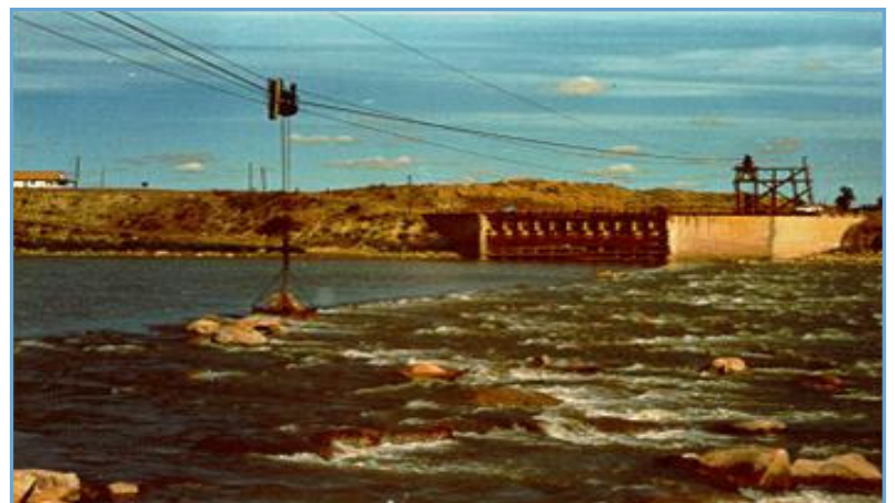
Historic photograph showing replacement of rock on Intake Diversion Dam
