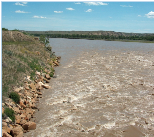
Yellowstone River flow along riprapped bank downstream from Intake
