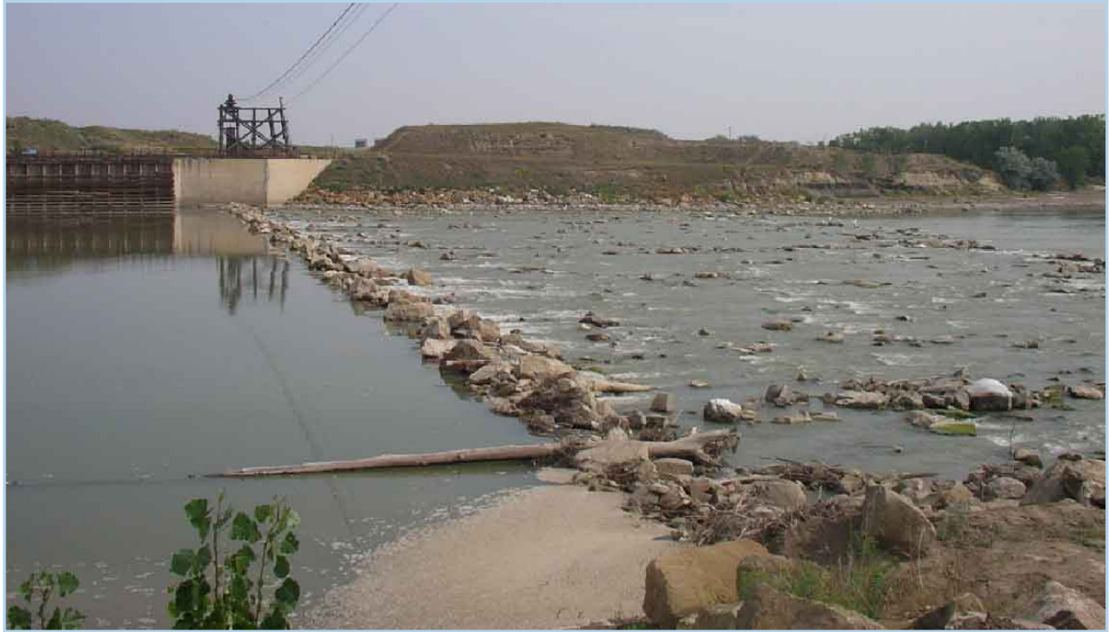
Intake Diversion Dam impedes fish passage on the lower Yellowstone River
