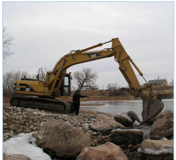
Construction of a rock ramp near Miles City, Montana (photo courtesy of Fish, Wildlife and Parks)
